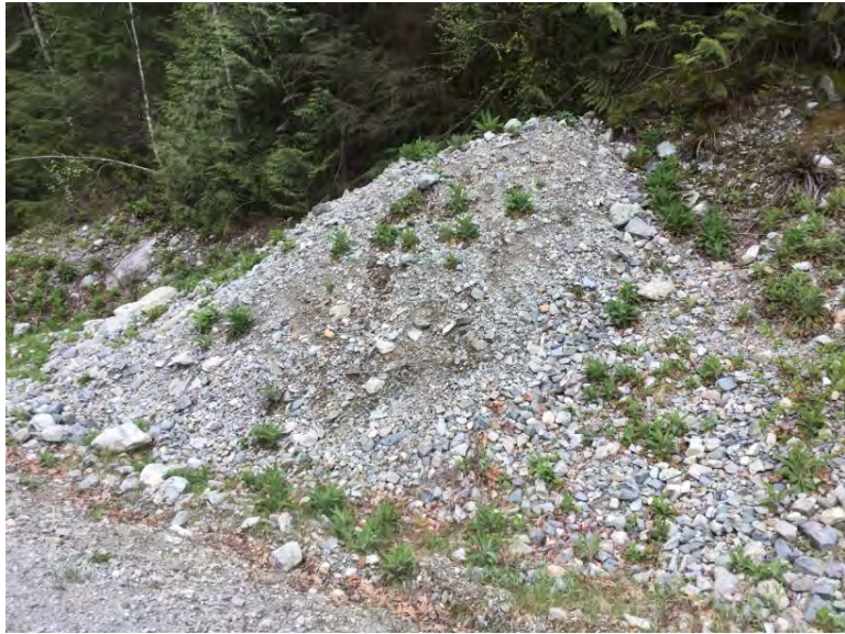
Inlet consistently being cleaned
